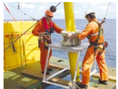
Buoyancy Module Installation
